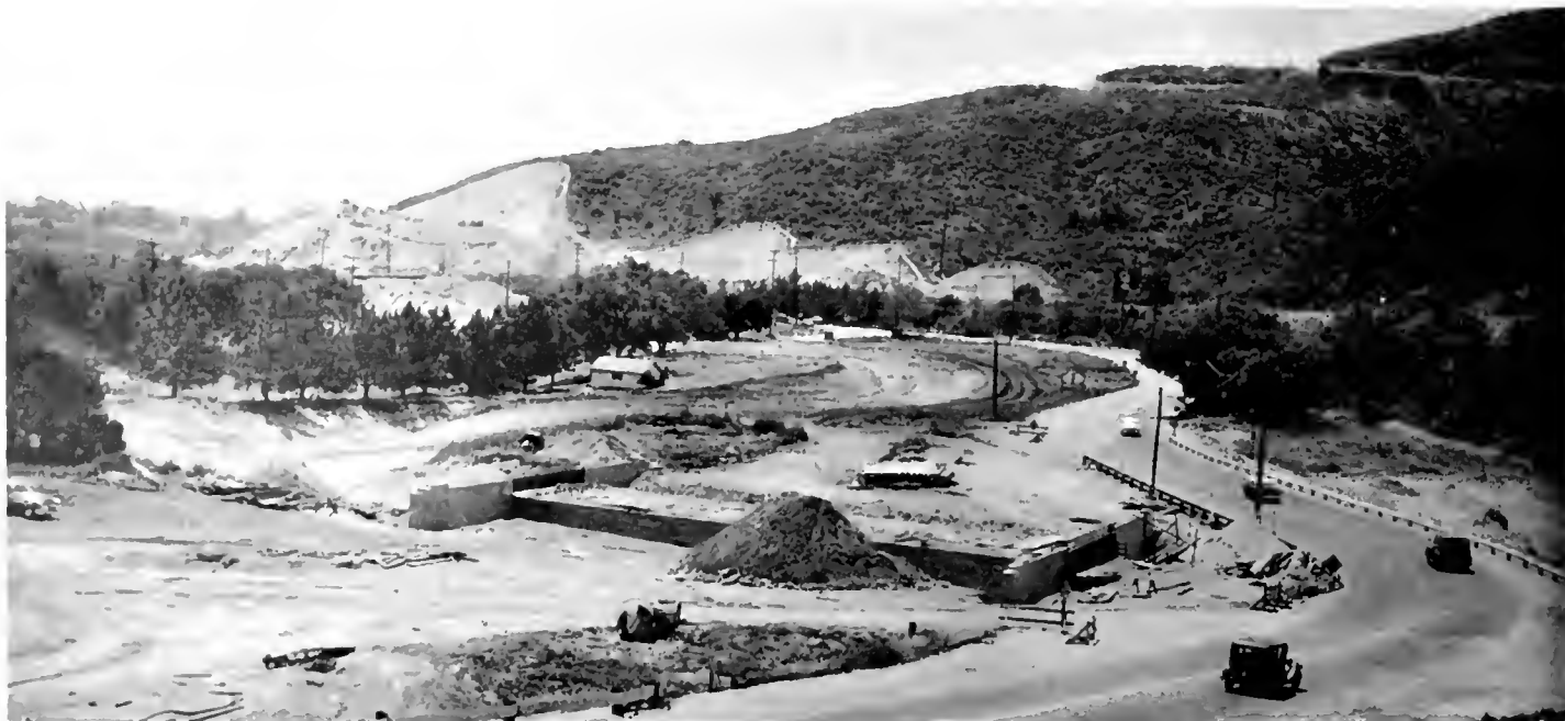
Looking south toward Highland Avenue cut. Structure in foreground is Berkshire Avenue Undercrossing which is substantially completed
